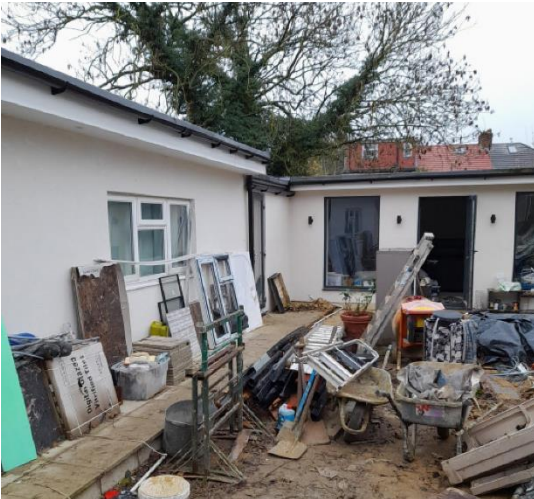
Office, corridor and gym/storage space at No.24
