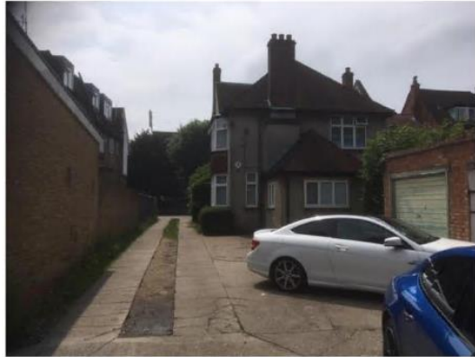
Rear of existing building facing High Road
