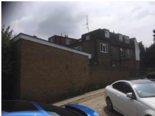
View from the site of adjacent buildings to the South
