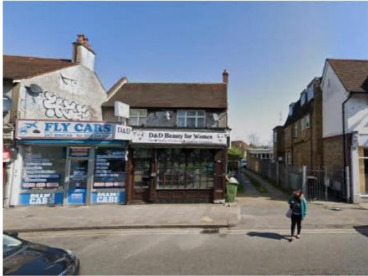
Site entrance and existing building facing High Road
